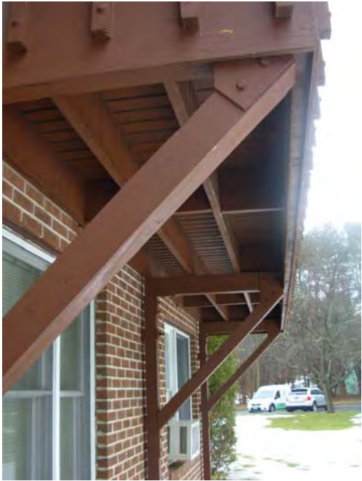
5. Supports added to balconies for more support
