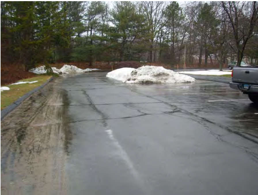
1. Parking surfaces display cracking and some settlement
