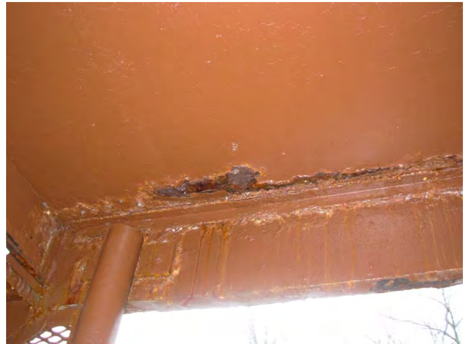
10. Egress stairway deterioration and rusting
