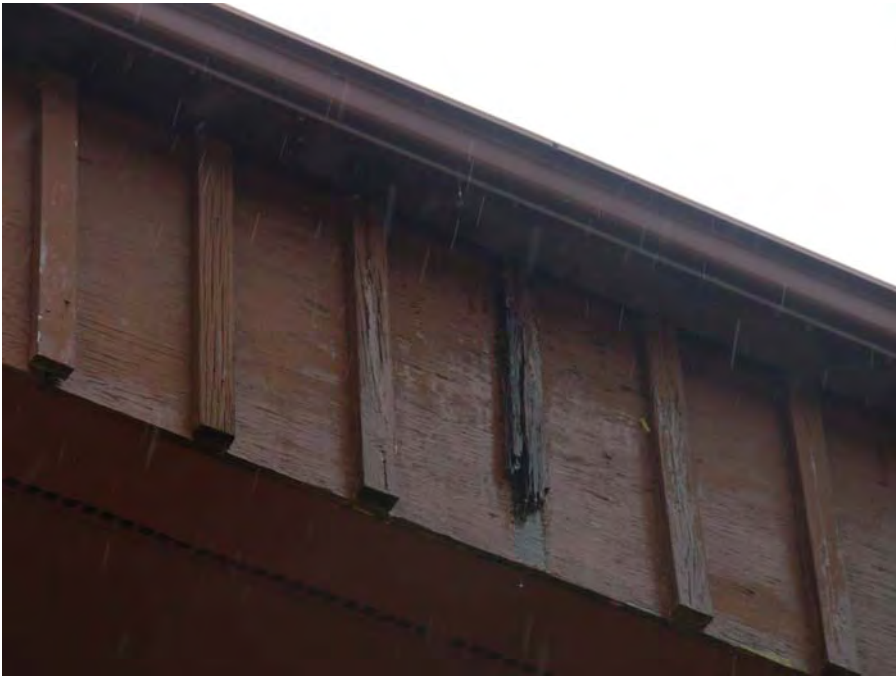
7. Trim element deterioration at fascias
