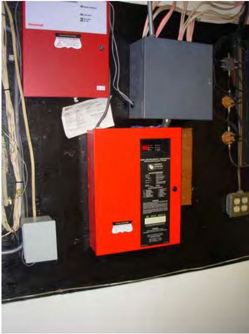
17. Fire detection and emergency call system monitoring panels
