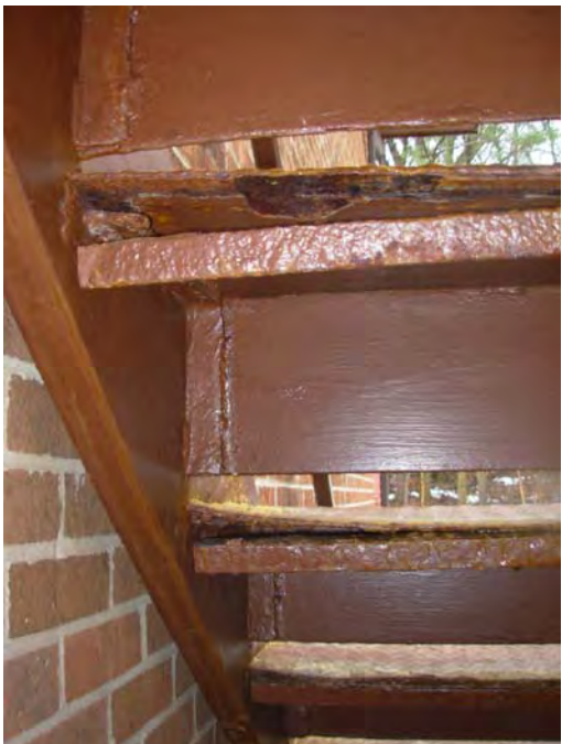
11. Egress stairway tread rusting and deterioration
