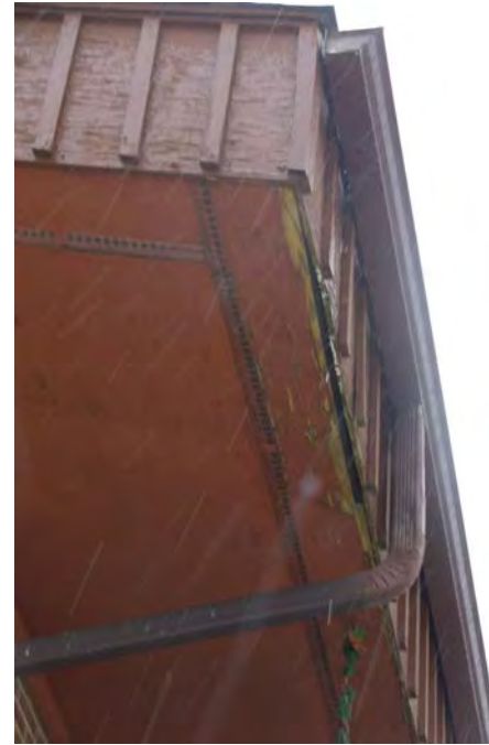
6. Soffit and fascia wood deterioration
